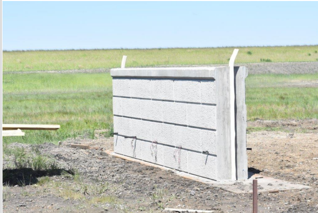
Sample Panel for Walls – Diversion Inlet Structure
